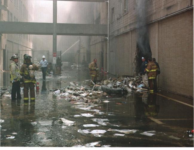
Above: In A-E Drive, debris and airplane tire remnant. Below: The "punch out" hole in A-E Drive.
