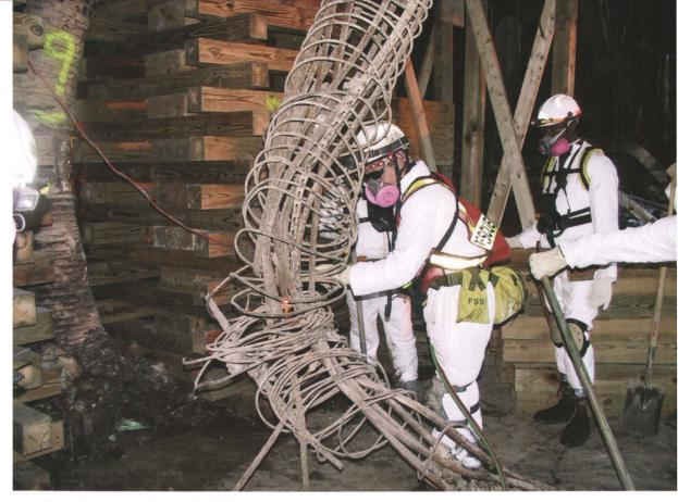
Above: Removing a damaged building column.
